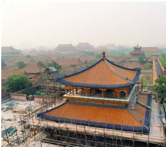
The Pavilion of Prolonged Spring under construction in the Forbidden City
